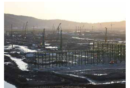
TPAO Natural Gas Processing Plant Zonguldak
